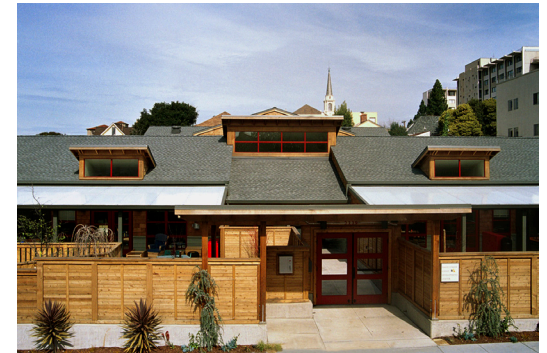
Using drought-resistant plants and mulch reduces landscape irrigation by 61% per LEED guidelines. Photo: Jonathan Martin.
