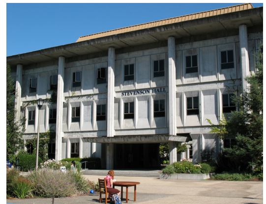
Stevenson Hall is slated to receive extensive lighting retrofits. Photo: Trista Little.
