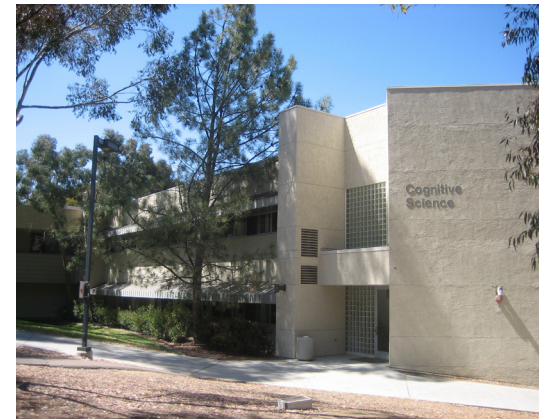
HVAC upgrades have cut the Cognitive Science building's energy use in half. Photo: John Dillio.
