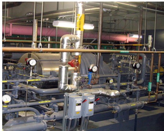
View of the steam turbine electrical generator (silver, foreground). Photo: John Dillio.
