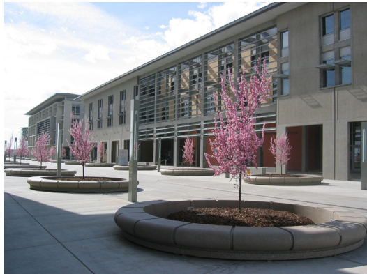
The Classroom and Office Building is UC Merced's second LEED Gold project. Photo: Michael Romano.
