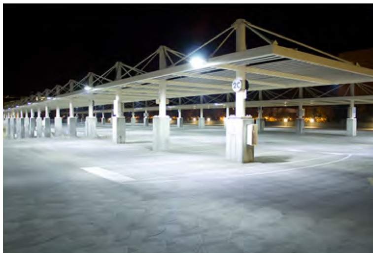
View of parking structure during off-peak hours. Photo: CLTC
