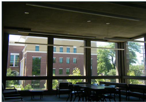
Daylighting sensors turn off pendant lights in corner reading areas when light is sufficient. Image: CSU Chico.
