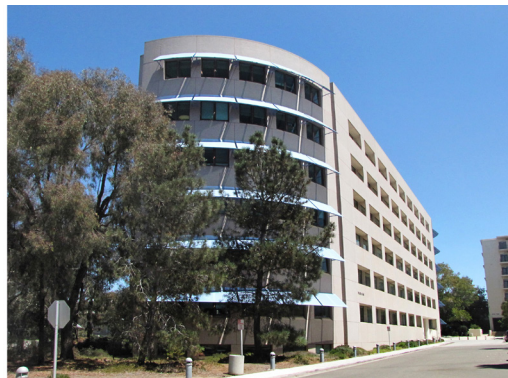
An HVAC retrofit at Pacific Hall yielded substantial energy savings. Photo: Rhett S. Miller, UC Regents.
