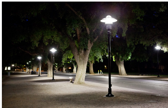
Lighting along pedestrian and bike paths retrofitted with dimmable LEDs that respond to users’ direction of travel. Photo: Kathreen Fontecha, CLTC/UC Davis.
