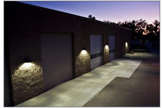
UC Davis campus dimmable LED wall packs. Photo: Kathreen Fontecha, CLTC/UC Davis.
