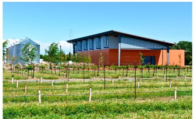
Exterior with window shading, water storage tanks, and overhangs on east and west exposures. Photo: Jasper Sanidad.
