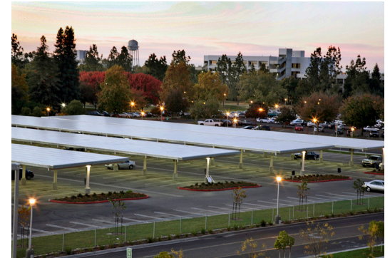
The solar canopies provide the only shaded parking on campus. Photo: Randy Vaughn-Dotta.
