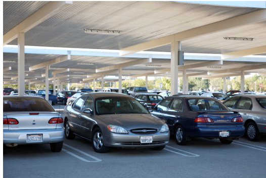
A corrugated aluminum covering protects cars from nesting pigeons. Photo: Randy Vaughn-Dotta.
