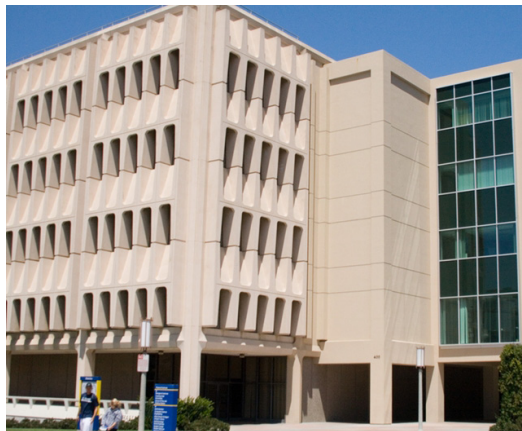
Constructed in 1968, Rowland Hall was in need of a massive replacement of air delivery systems. Photo: Matt Gudorf.
