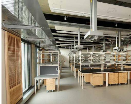
*Laboratory interior shows upper daylight glazing and lower glazing with sliding louver panels. Photo: Lara Swimmer Photography.*
