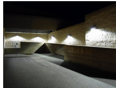
Before and after installing bi-level LED wall-pack fixtures. Images: Andy Shatney.
