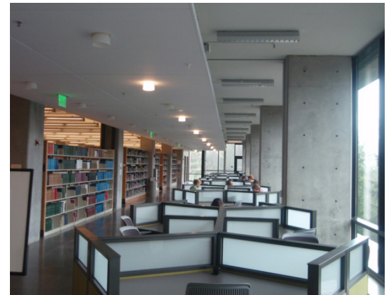
Perimeter in McHenry Library after delamping and retrofitting controls. Image: Andy Shatney.
