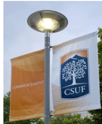
New LED pedestrian fixture at CSUF. Image: Doug Kind.
