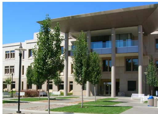
The HVAC retrofit of the PES lab will yield significant energy savings. Image: UC Davis.
